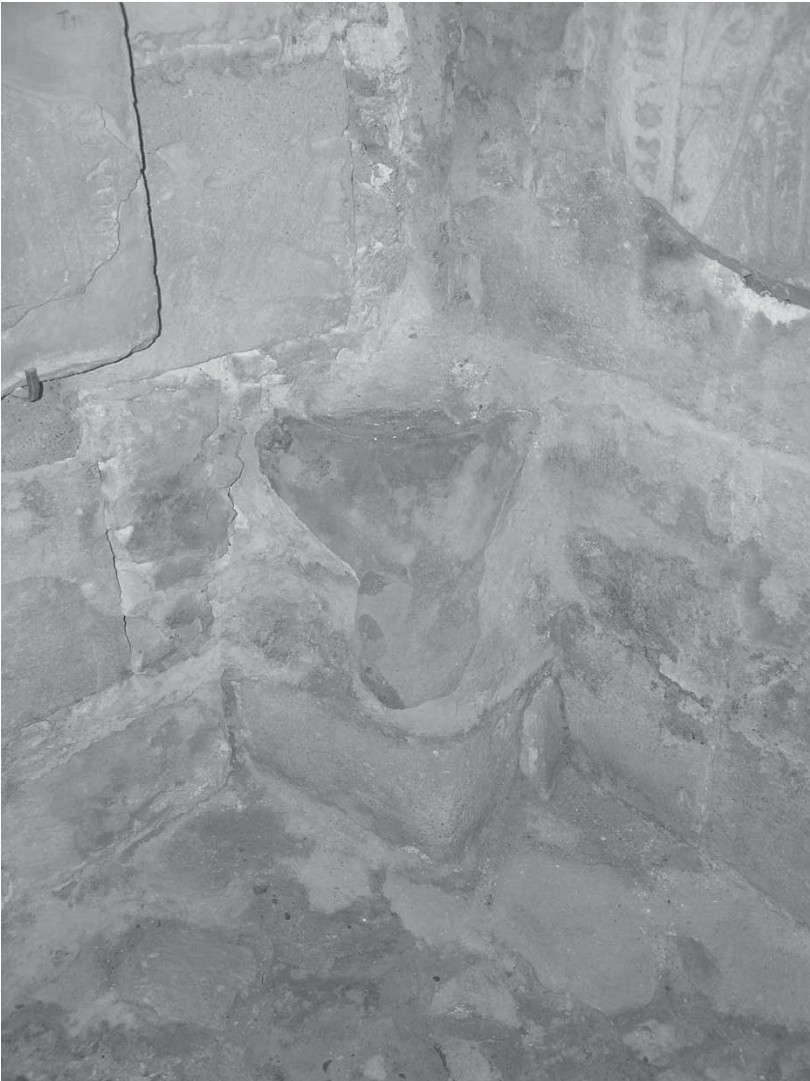
Fig. 20: Limassol Castle, cellars, east wall, detail of apse respond base and plinth [M. Olympios].
